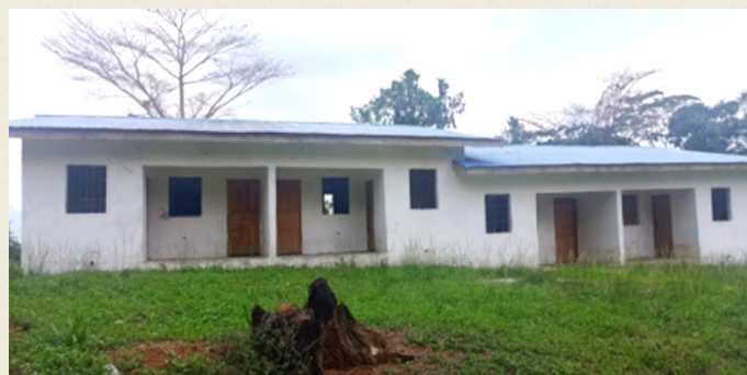
An incomplete teacher’s quarter constructed by Solway in Gbarpa. © CS-IFM
