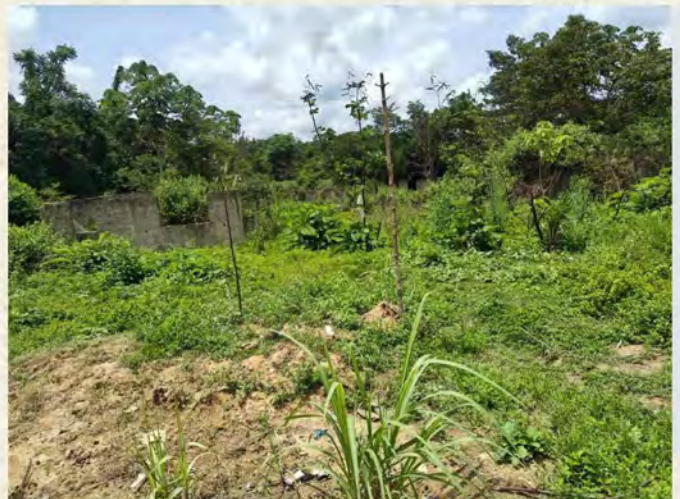
@SDI - Gbalawein school construction abandoned by Mandra
