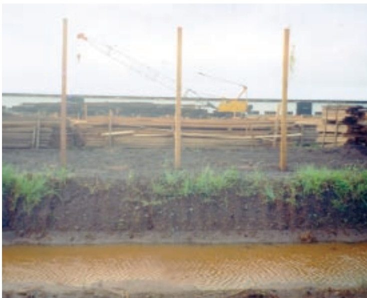
OTC's unfinished plywood mill, Buchanan; July 2001
