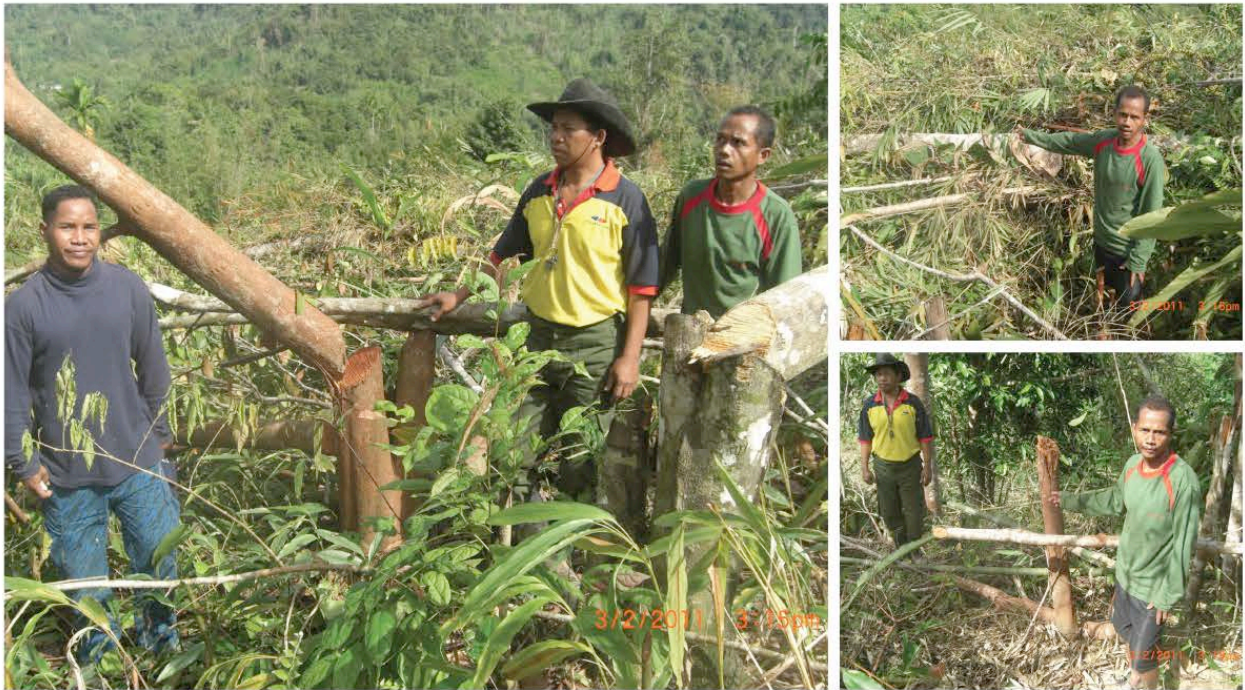
The construction of a workers' accommodation facility for a plantation project destroyed the farms, orchards and burial ground of the community in February 2011.
